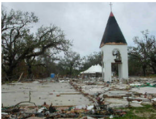
In the Diocese of Mississippi, seven Episcopal Churches were totally destroyed. This photo shows what was left of Christ Episcopal Church, Bay St. Louis. The stones (inscribed with deceased parishioners names) in the Memorial Garden lay haphazardly on the ground.
